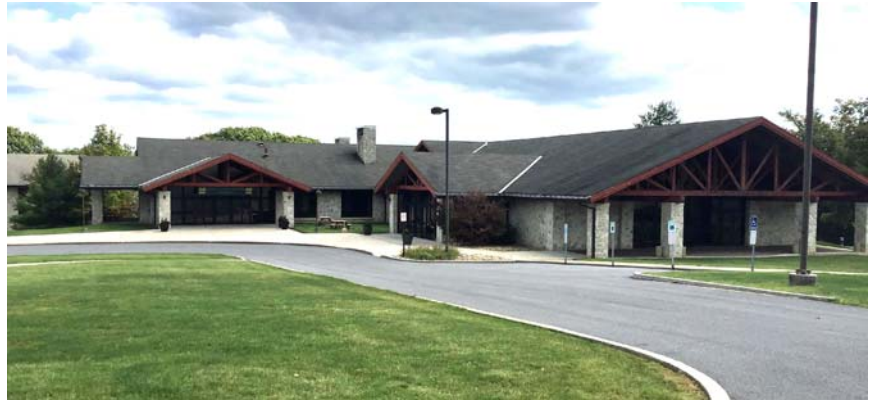
Conference Center at the Living-Learning Center, University of Pittsburgh - Johnstown. Parking is in the lots to the left (north). S. Lindberg photo
